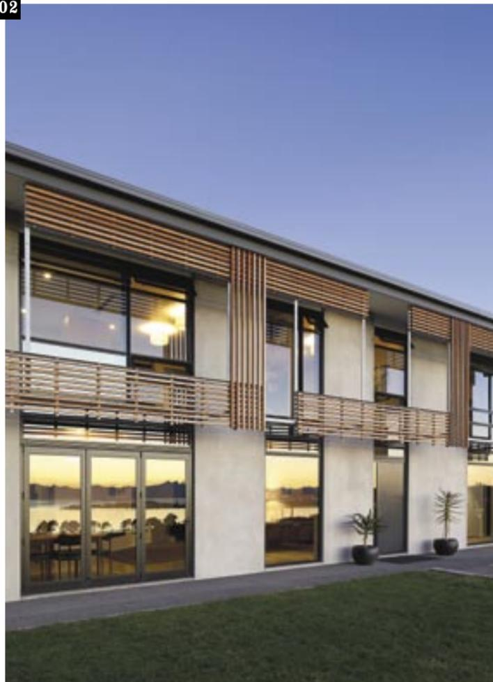
Architects often explore and exploit the boundaries emplaced by the restrictions of building, and Jeremy Smith has followed suit through the design of the Tilt Panel House. Concrete tilt panel construction, which is often a commercial approach to fabricating buildings, was used by Smith as a way to provide a durable, cost efficient and thermally sustainable solution for the four bedroom family house on a new suburban subdivision in Nelson.
